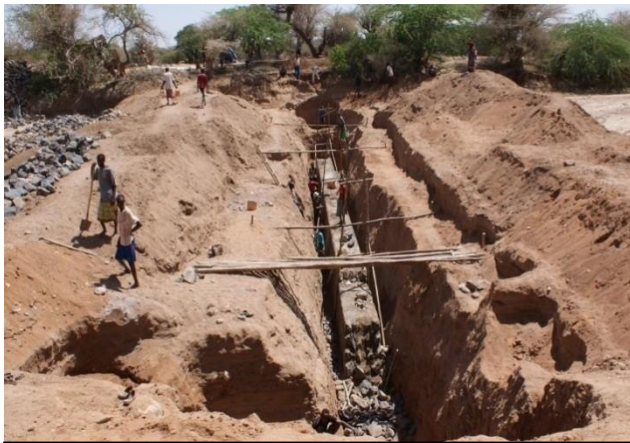
(a) Construction of Subsurface dam
