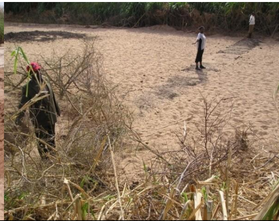
(b) subsurface dam just after construction
